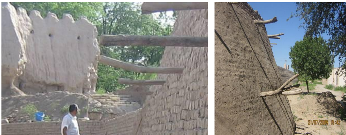
3-Fig. The use of timbers on the wall of the Deshon kala monument
