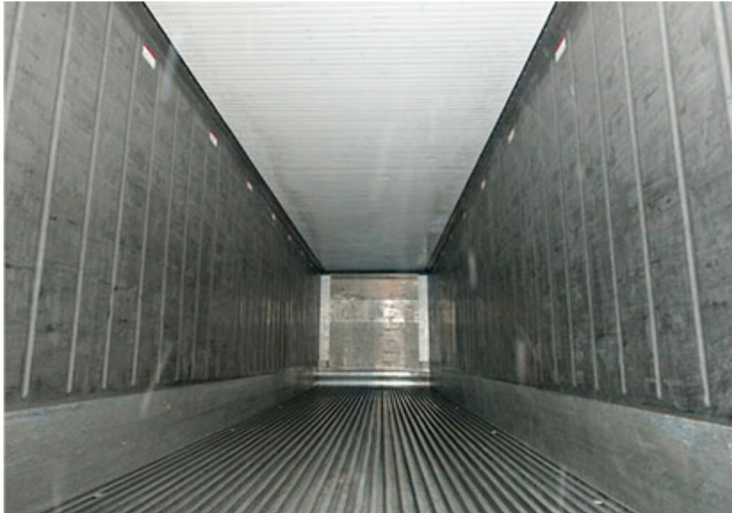
Figure 14. Ceiling structure of a 40-foot refrigerated container.
