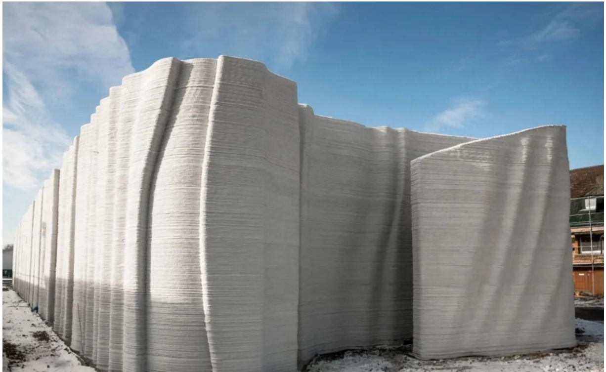
Figure 6. The largest 3D-printed structure in Europe [9].
