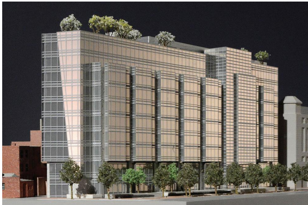
Figure 5. A typical 3D printing building [8].
