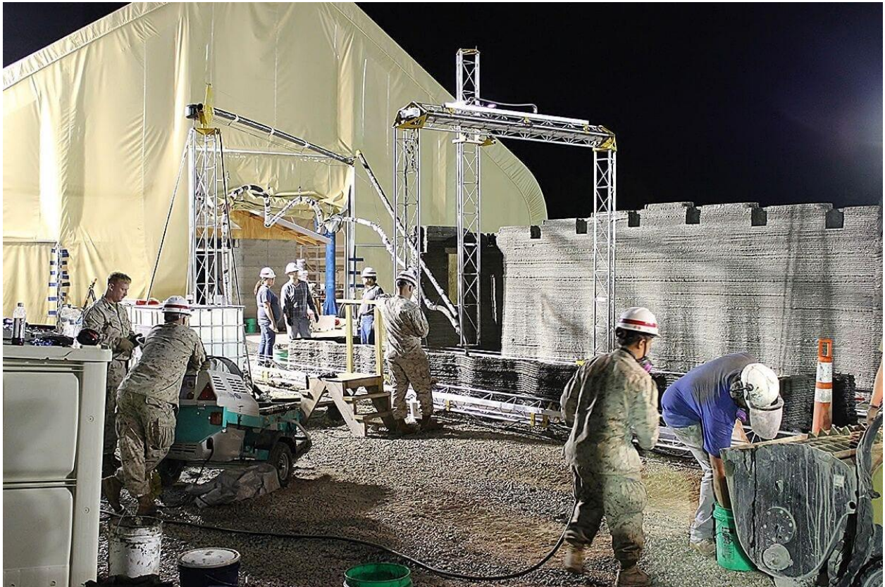
Figure 1 World's largest concrete 3D printer constructs barracks [1].
