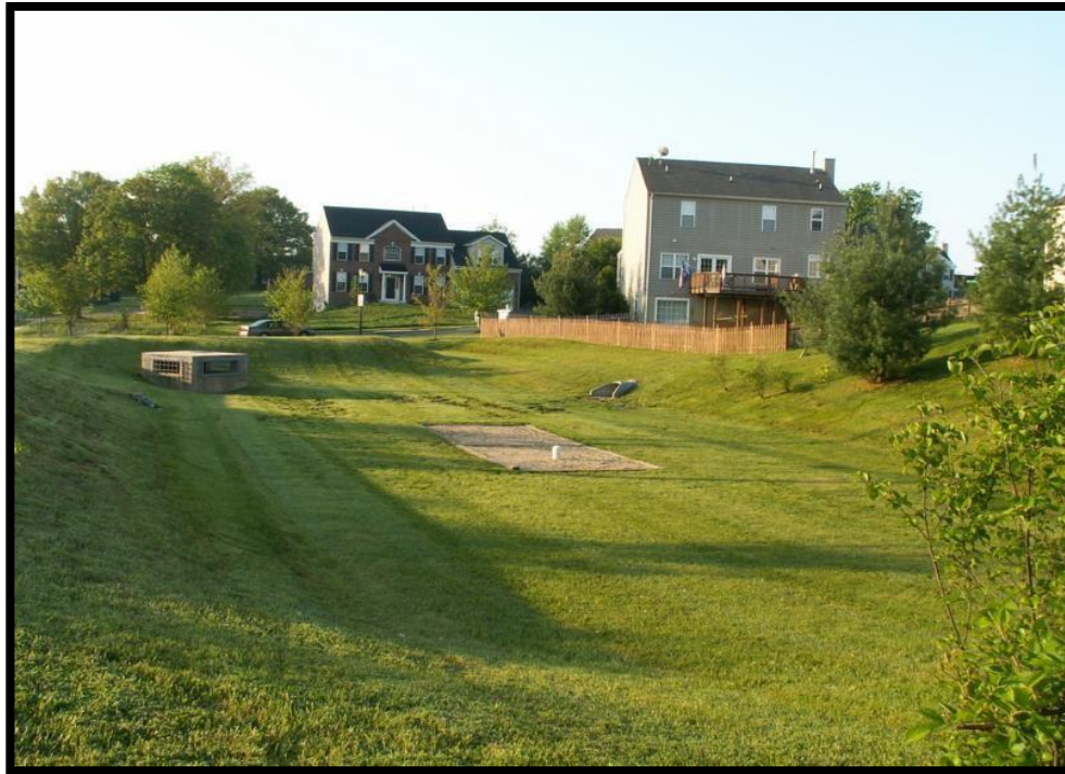
Figure (5) Detention pond
