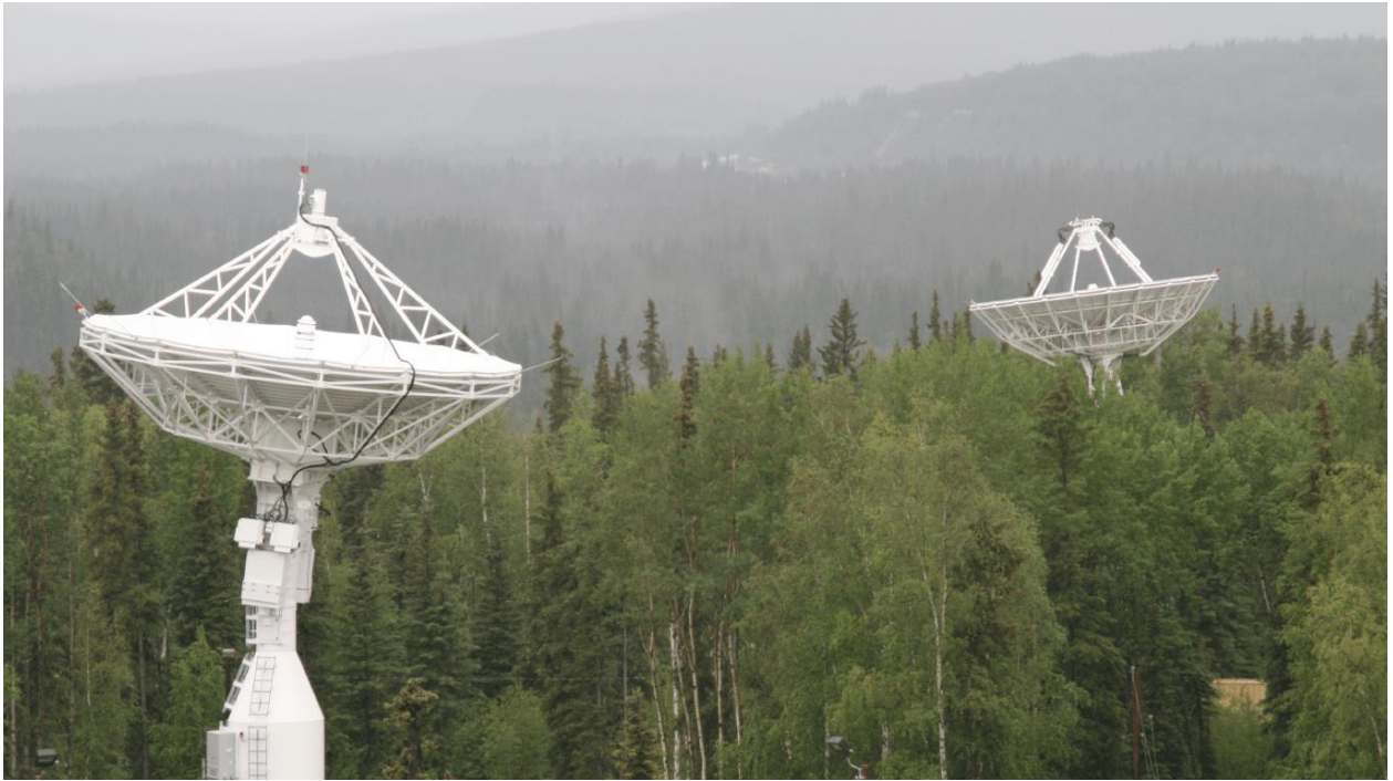
Figure 6. Two ground antennas located in Fairbanks, Alaska [6].
