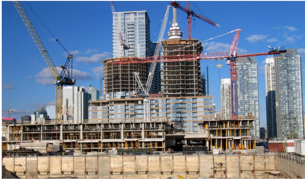
Figure 6. A typical construction site [9].
