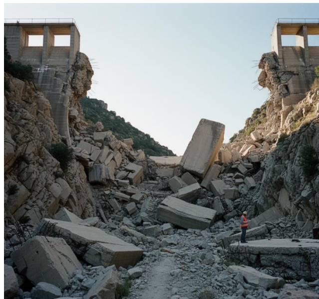
Figure 2. Aftermath of the Malpasset Dam failure (1959)
